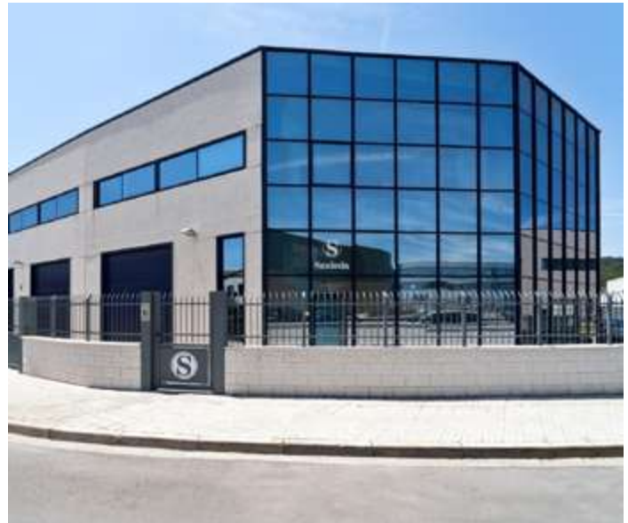
Logistic platform. Malgrat de Mar, Barcelona.
