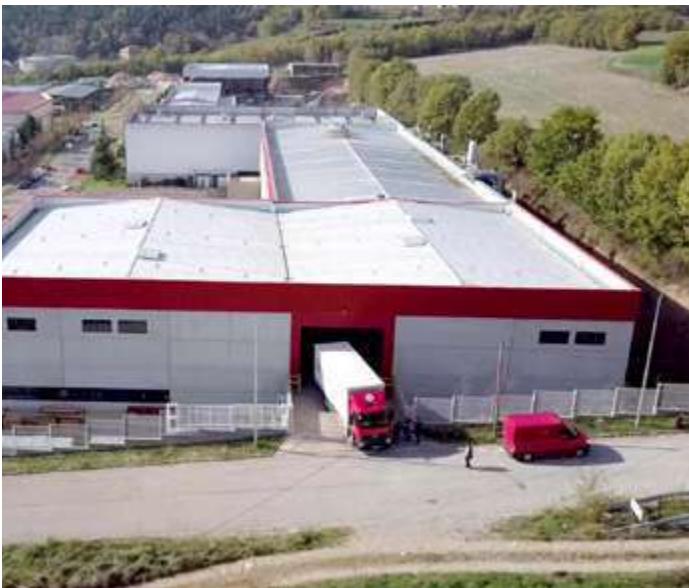
Technical textiles plant. Berga, Barcelona.
